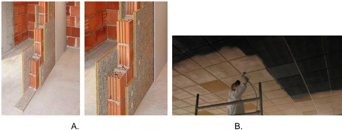
Figure 6 Application of Heraklith panel with stone wool as heat and sound insulation, and fireproof material on the surface of bricket wall; B: Ceiling and painting application of Heraklith panel
