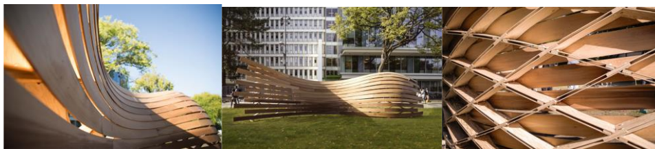
Figure 9 Wooden structures as a product of digital design and implementation: Timber Wave prototype, doubly curved timber assembly, at the University of British Columbia Campus (Correa et al., 2019)
