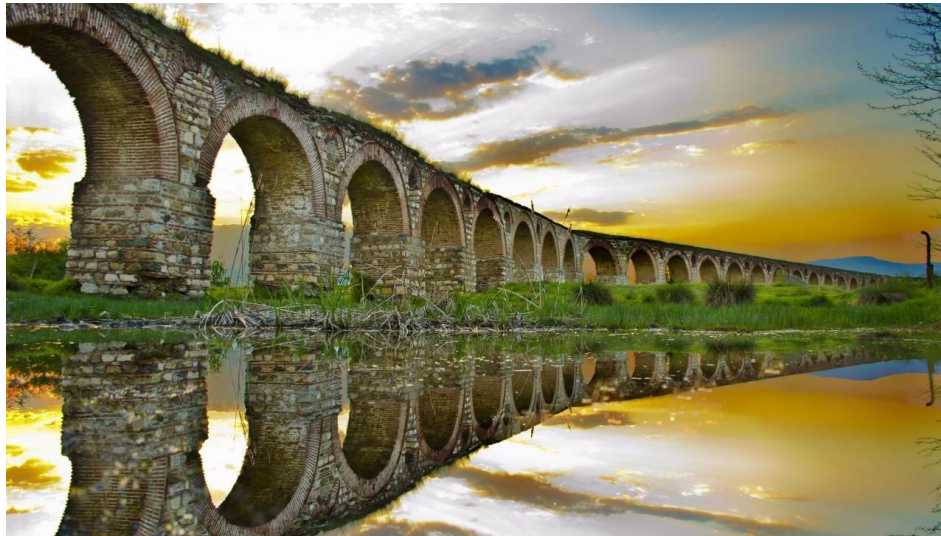
Figure 1 View on the Skopje Aqueduct
