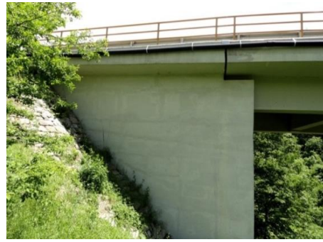
Fig. 2.2. View of one abutment of the chosen representative bridge
