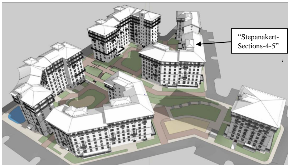
Fig. 1 Design view of the residential complex consisting of 9- and 7- story base isolated buildings to be constructed in the city of Stepanakert in 2020
