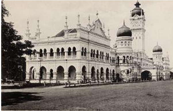
Figure 1. Sultan Abdul Samad Building in 1920
